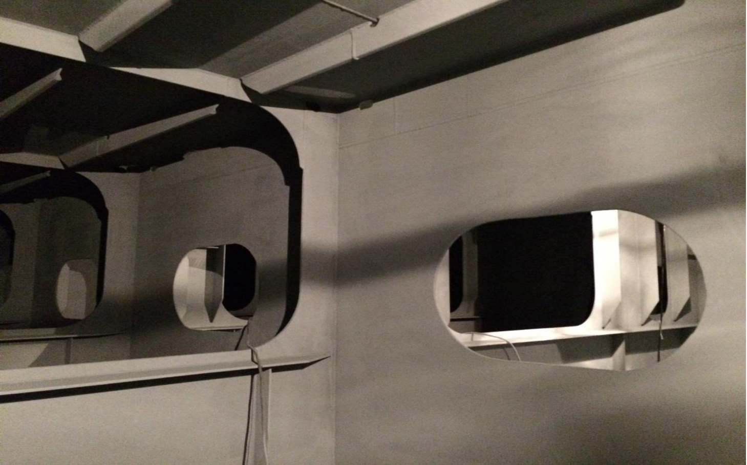
Methanol storage tank painted with zinc silicate
