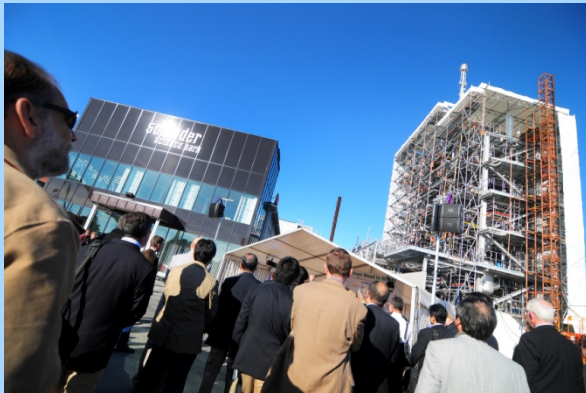
CHEMREC pilot plant in Sweden (4 t/day Bio-DME)
